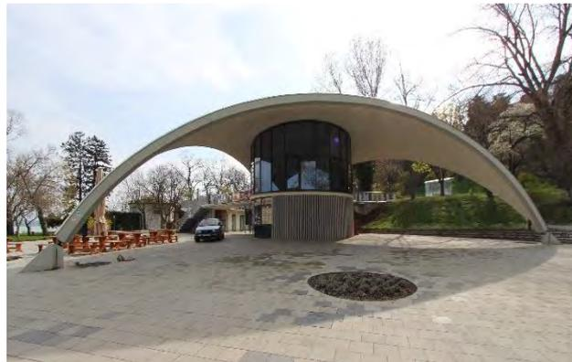
**Fig. 4** Reinforced concrete shell after the rehabilitation (2018, Tihany).
