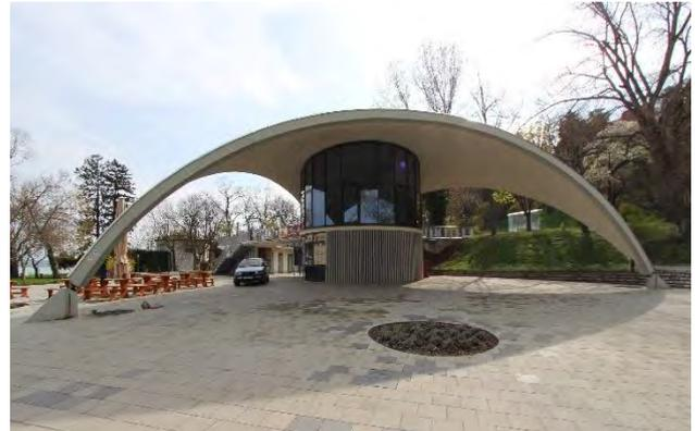
**Fig. 4** Reinforced concrete shell after the rehabilitation (2018, Tihany).
