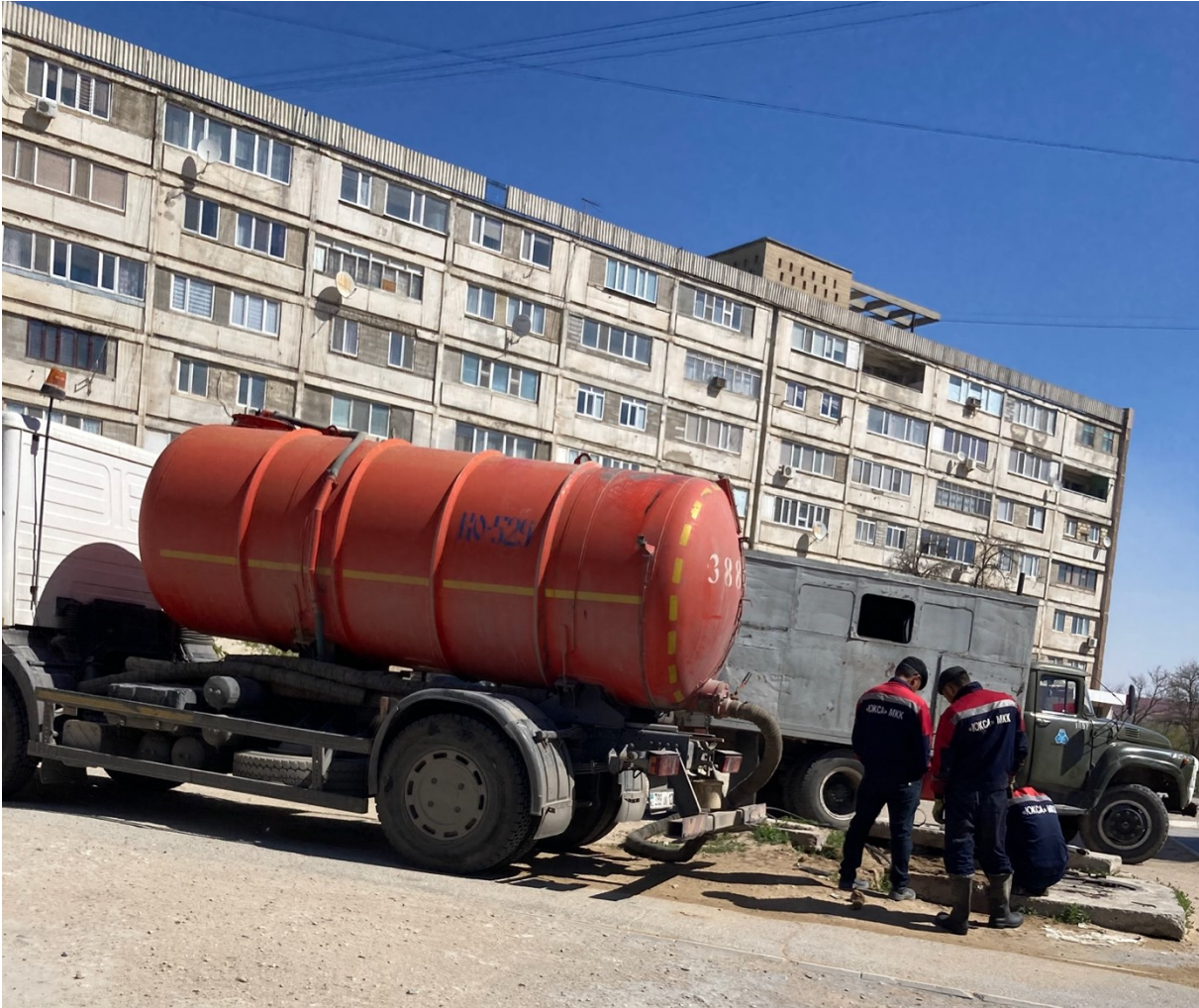
Figure 3. The 4th neighbourhood, Aktau, repairing the breakage. Taken by the author
