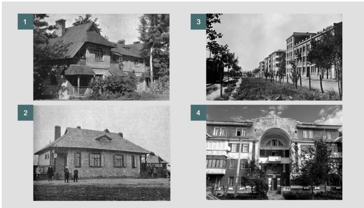
Figure 3. Photos of houses in workers' settlements of Kharkiv. 1. Residential building of the Kharkiv Locomotive Plant. (Source: from the book Essays on the history of architecture of the Ukrainian SSR, 1962 ). 2. Residential building in the Red October settlement (Source: From the archive of M. Kornilov). 3. Red Ray settlement (Source: From the archive of M. Kornilov). 4. Residential building of Machine builders settlements (Source: Authors).
